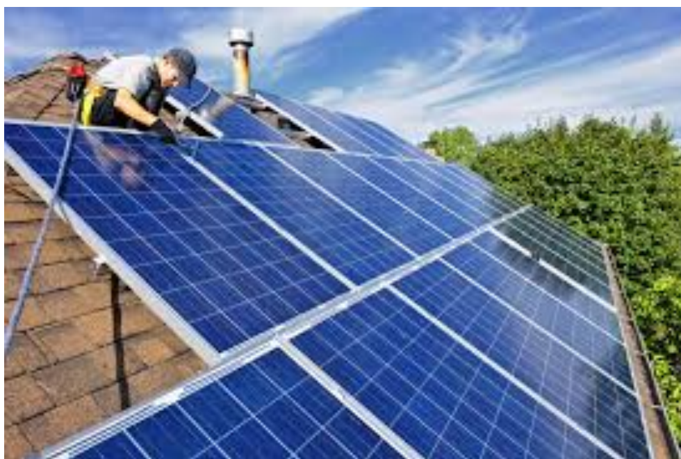
Figure 5. Behind-the-meter, rooftop solar has recently tipped 5 GW in installed capacity in Australia
