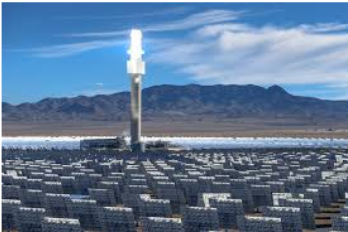
Figure 2. Crescent dunes in Nevada U.S. uses 10,347 heliostats to heat molten salt producing 1.1 GWh of energy storage
