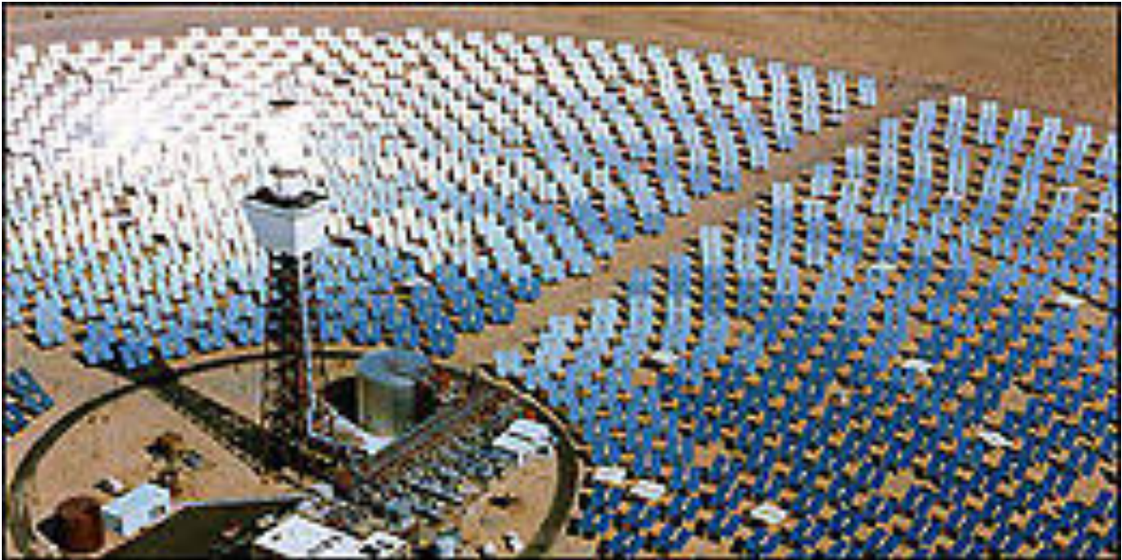
Figure 4 typical surround layout of heliostat field
