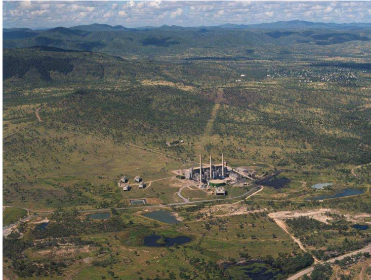
Collinsville Power Station – 180MW, coal-fired
