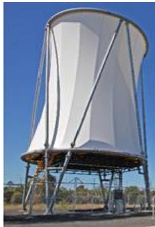
**Figure 4.23 – UQ Gatton tower (sized to cool a 1-MWe sCO<sub>2</sub> power block)**
