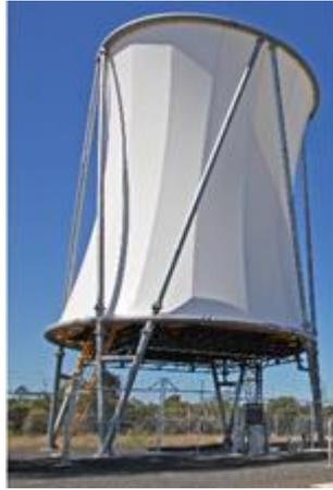
Figure 4.46 – UQ Gatton tower (sized to cool a 1-MWe sCO<sub>2</sub> power block)
