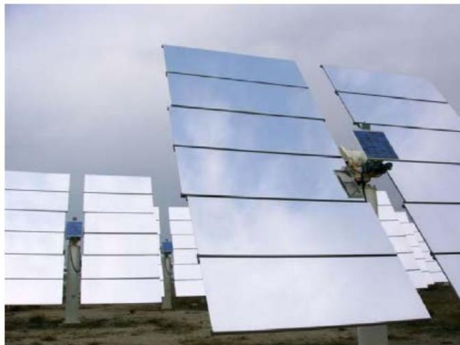
**Figure 46. A view of the PSA CRS heliostat field, which has 92 autonomous radio-controlled units.**
