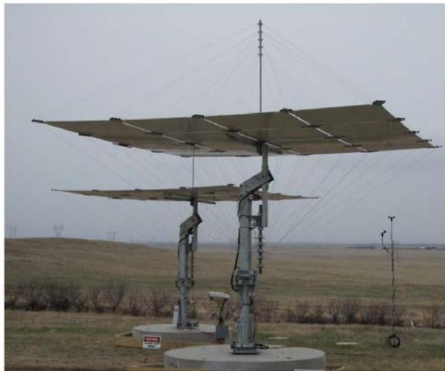
**Figure 6. Solaflect's 16 m<sup>2</sup> 'suspension heliostat' [26]**
