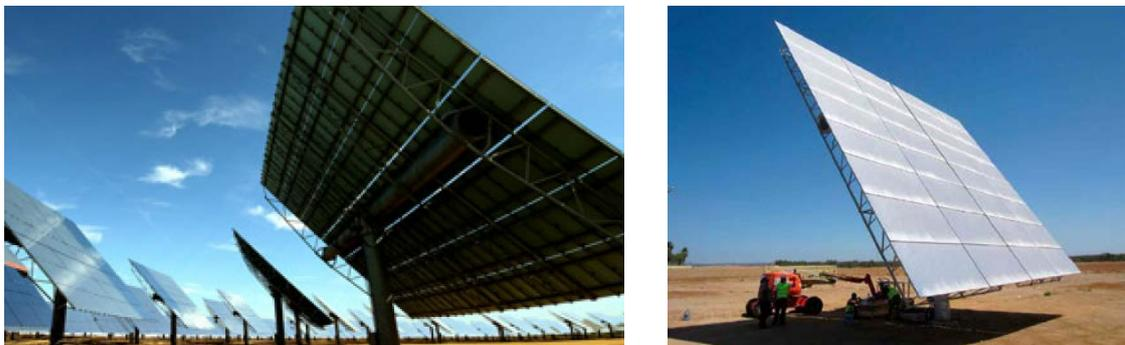
Figure 3. Abengoa Solar heliostats – the Sanlúcar 120 (left) [19] and the ASUP 140 (right) [21].
