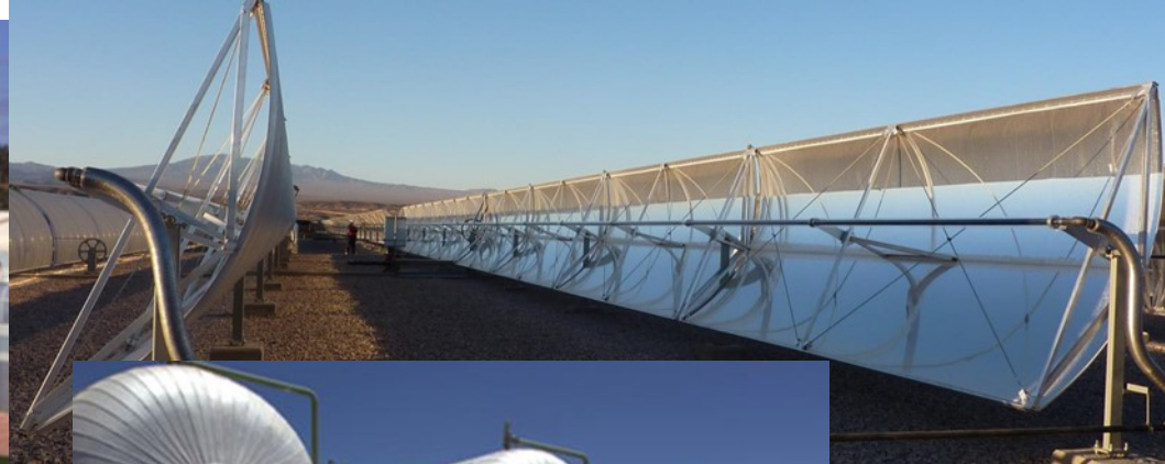
10MW th solar thermal trough array for 250°C, at a copper mine in the Atacama Desert Chile.
