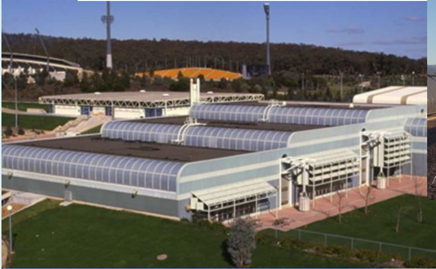
AIS aquatic centre, 1,500m 2 of unglazed collector
