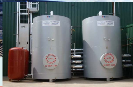
De Bortoli winery Griffith NSW, 100 x 30 tube collectors to deliver 12,000L of water per day, at 95°C
