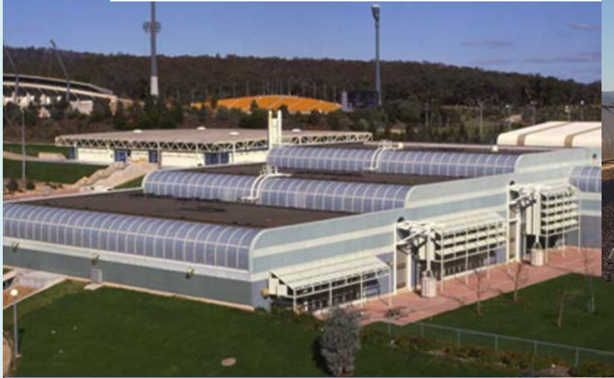
AIS aquatic centre, 1,500m 2 of unglazed collector
